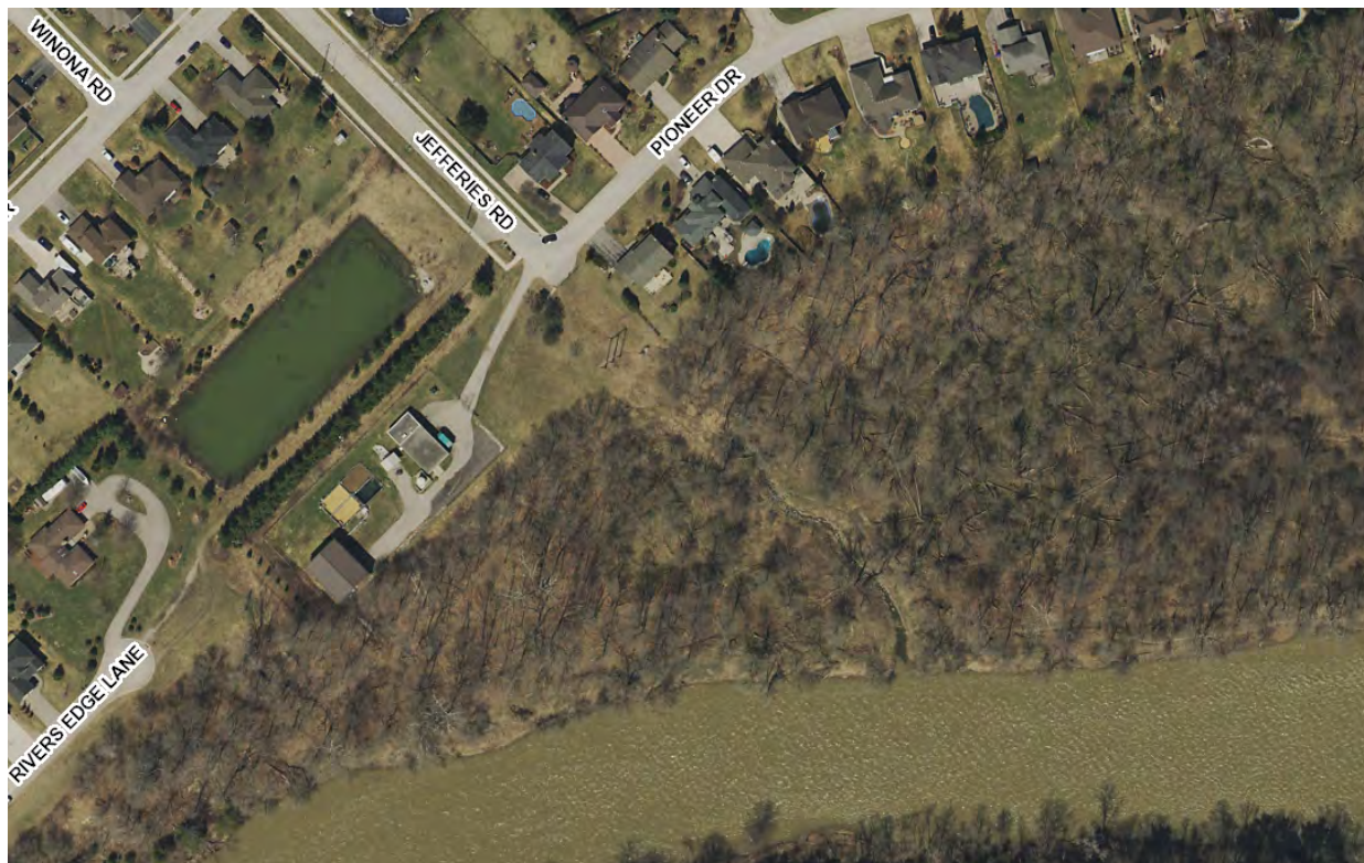
Figure 2: Jefferies Road Pump Station and Thames Riverbank
