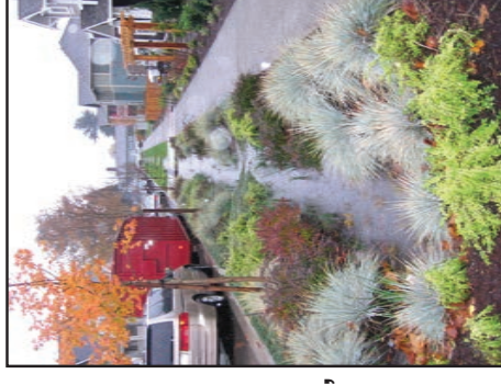
Example of a vegetated bioswale
