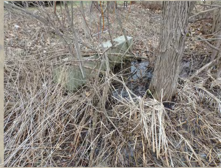
Photo 1 Ditch Inlet Catchbasin
