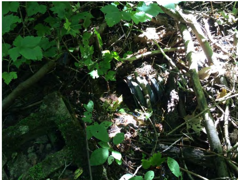
Photo 6, BigO drainage tile located along north side of Harris Road.
