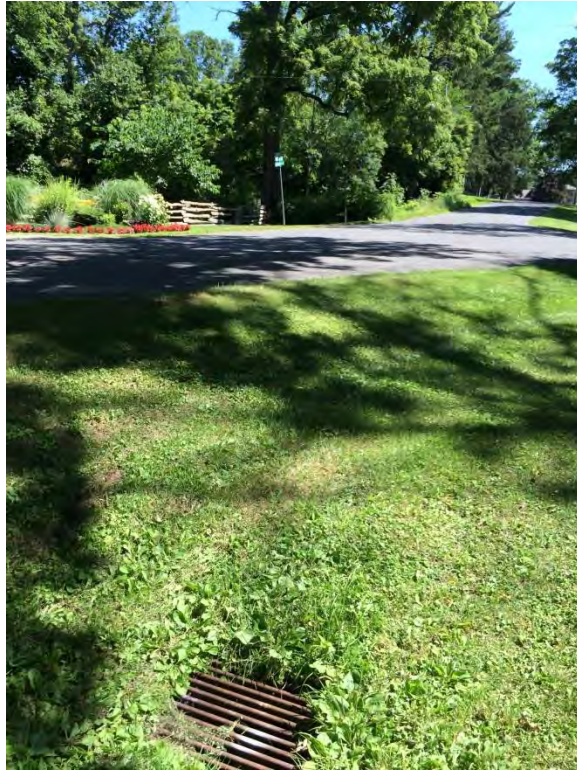
Photo 9, Inlet grate at intersection of Millcreek Lane and York Street.
