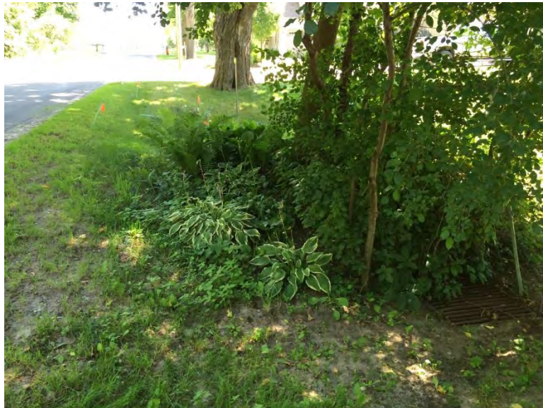
Photo 4, Inlet grate located along south side of Harris Road.
