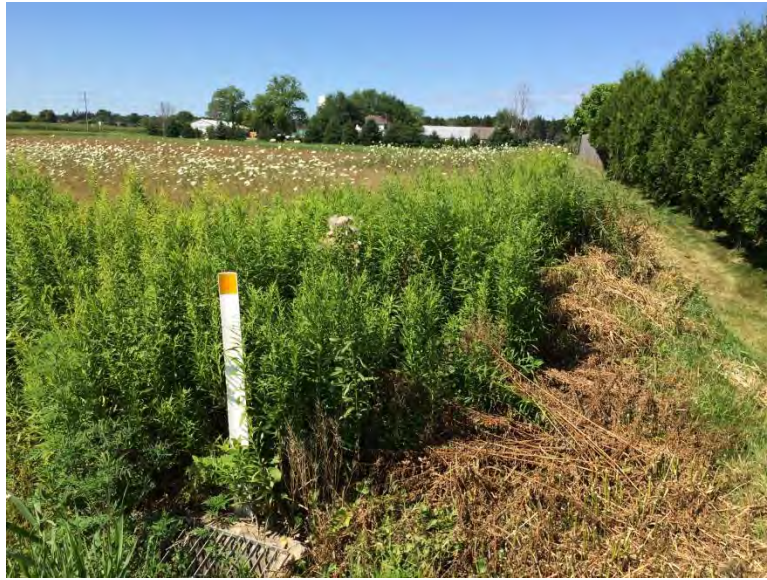
Photo 1, Beside grated inlet looking west at where Cummings Drain intersects with Martin Road.
