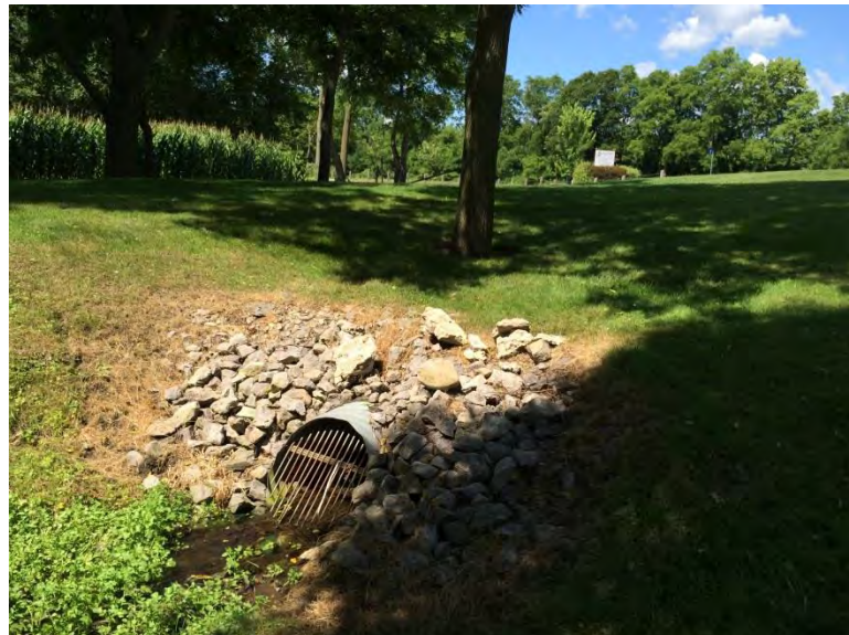
Photo 12, Pleasant Street Culvert.
