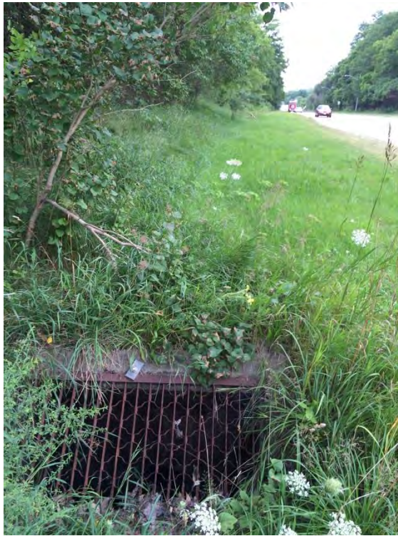
Photo 18, Inlet grate located along south side of Longwoods Road.
