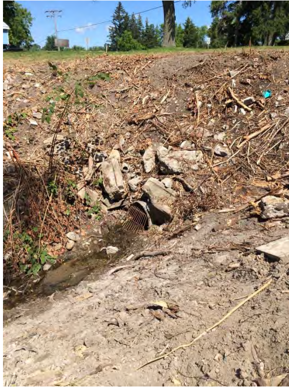
Photo 11, Outfall located along west side of Gideon Drive.
