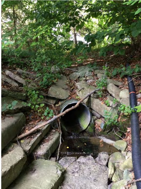
Photo 19, Outfall located along west side of Springer Road at William Street.
