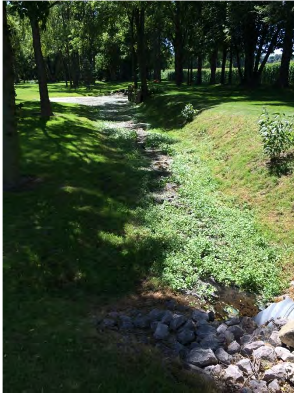
Photo 13, Looking south from Pleasant Street Culvert.
