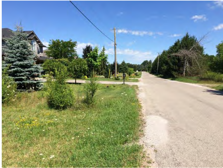
Photo 3, Drainage swale located along west side of Martin Road.
