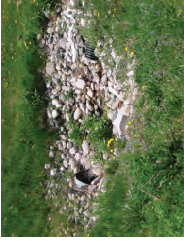
Pleasant Park Culverts
