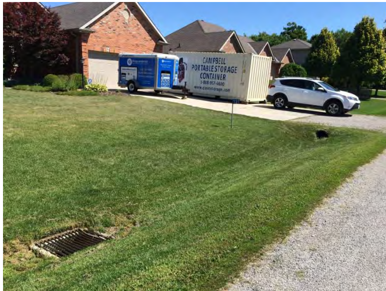
Photo 2, Inlet grate and drainage swale located along north side of Wellington Street.
