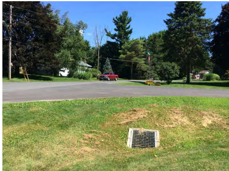
Photo 10, Inlet grate located at Yorkdale Street and Millcreek Lane.
