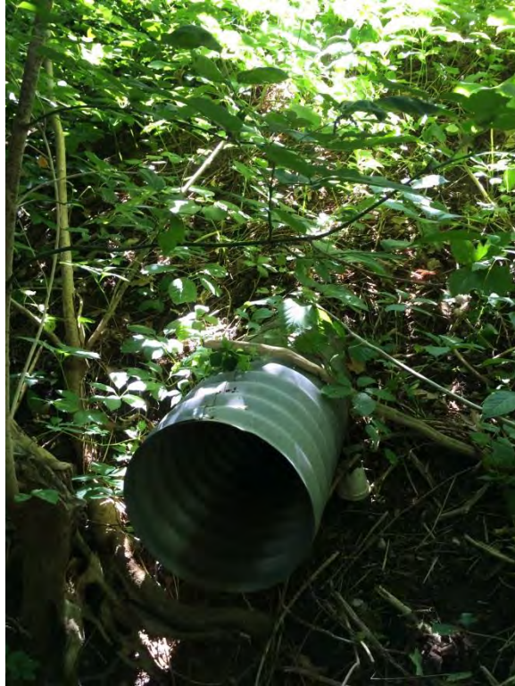
Photo 5, CSP outfall pipe located along north side of Harris Road.
