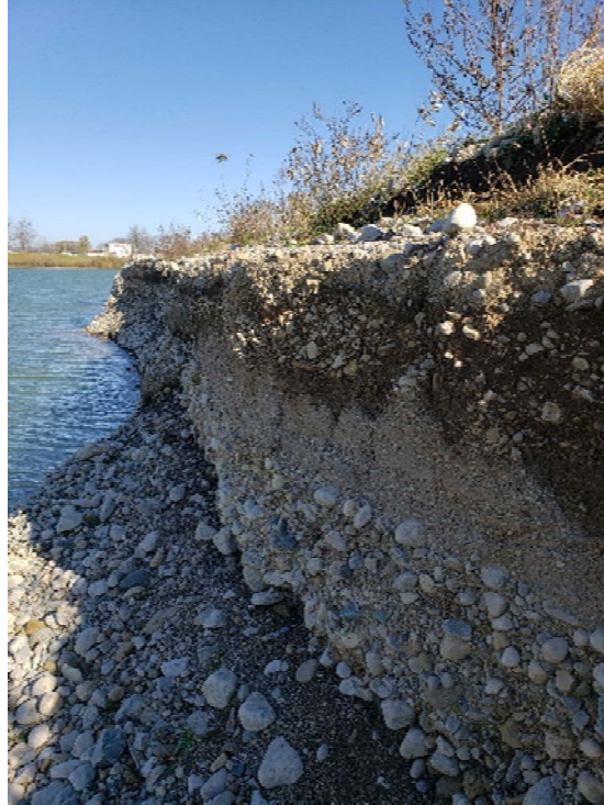
Figure 1: Exposed Aggregate at Current Limit of 30m Buffer Zone
