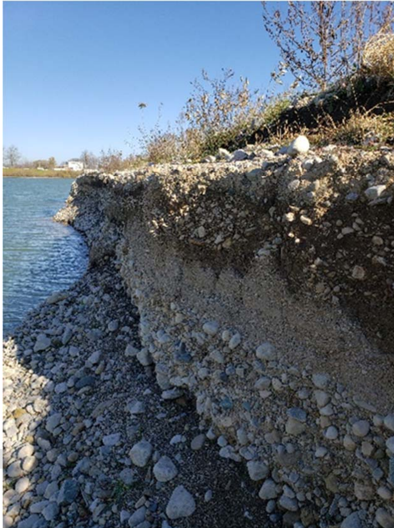
Figure 3: Exposed Aggregate at Current Limit of 30m Buffer Zone
