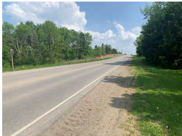
Photo 4: Disturbed area, showing municipal road ROW, facing south-southeast
