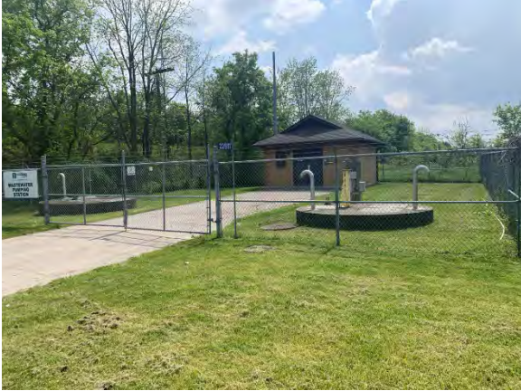
Photo 5: Disturbed area, show existing infrastructure, facing south
