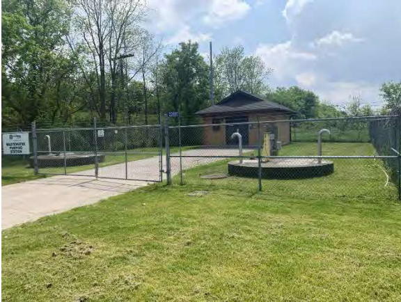
Photo 5: Disturbed area, show existing infrastructure, facing south
